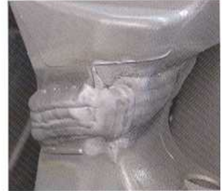
Welding beads with no wash applied.
